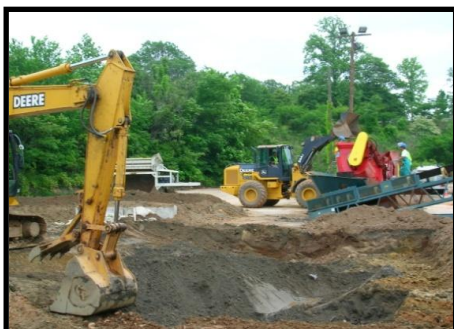
Former UST Pit/Area of Treatment
