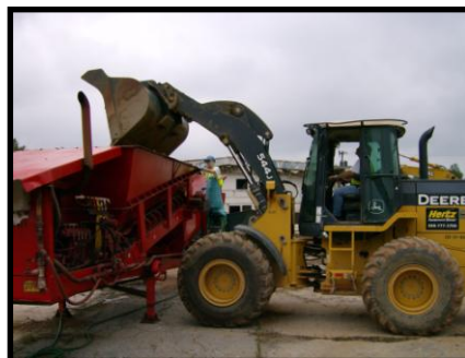
Placing Contaminated Soil into Auger-Driven Blender
