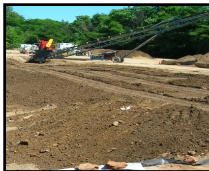
Completed Area after Backfilling of Clean Soil
