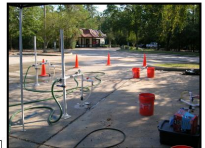
ISCO Injection of Klozur®
